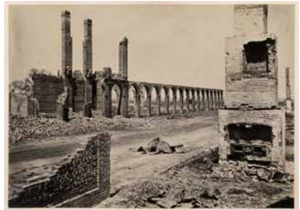
George N. BARNARD Ruins of the R.R. Depot in Charleston
